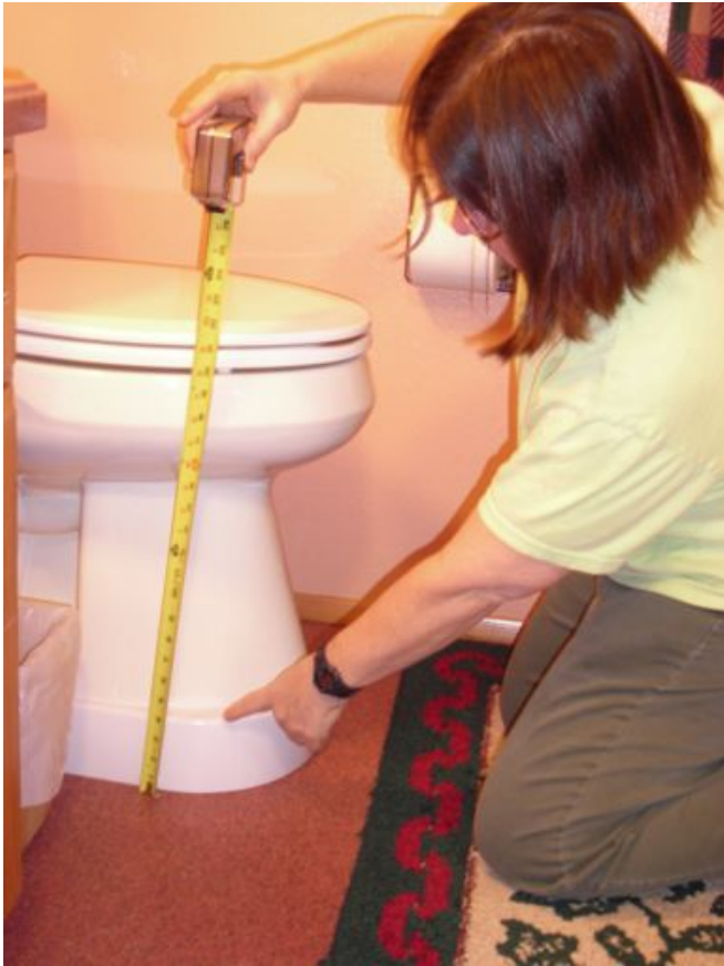
A Toilevator mounts under an existing fixture, adding ~4"
